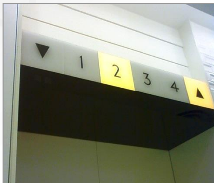
Illuminated Elevator Floor Display
